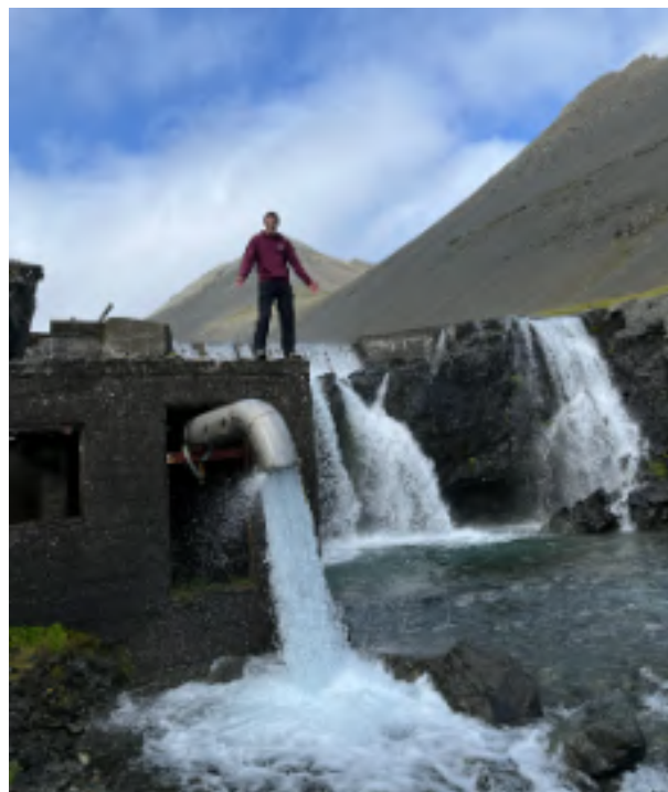
Figure (4.47) Strange plumbing filled building at the waterfall
